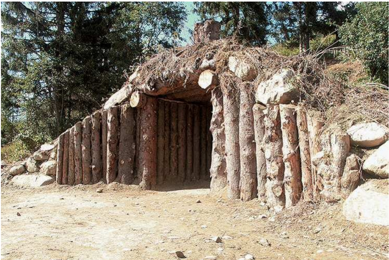
Roundwood shelter made of spruce and larch.
