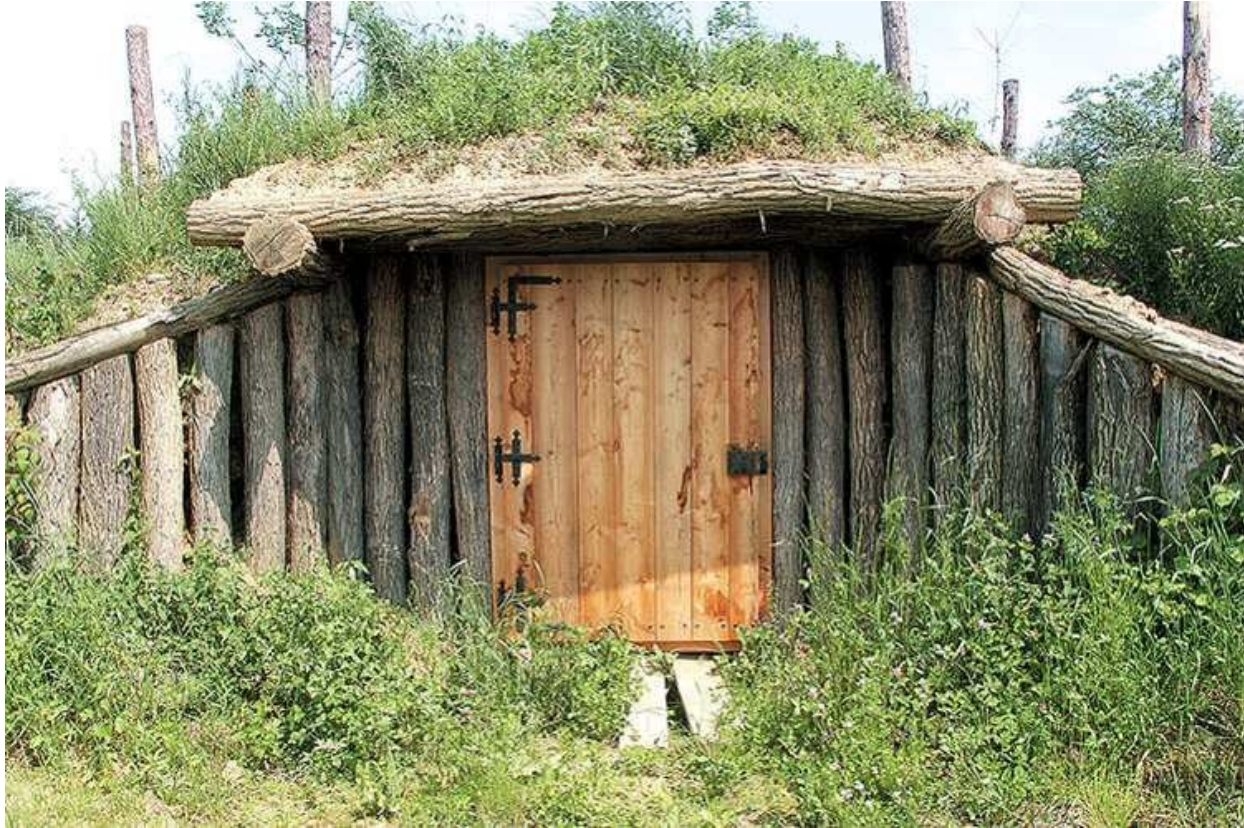
Storage room made from robinia logs.
