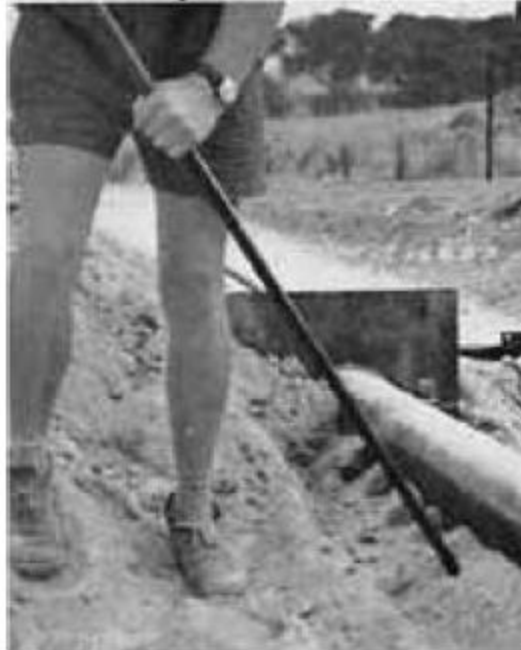
Plate 26 Ramming under the Lockpipe is very important.
