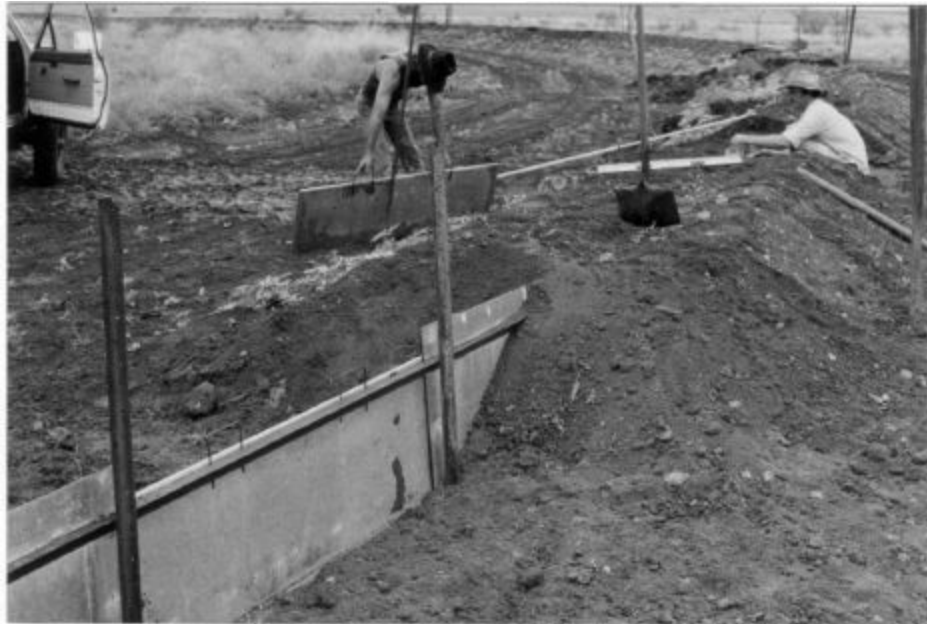
Plate 47 A newly positioned 1.2 m (4 feet) wide water gate supported by “star” steel posts. The opening panel slides in a slot formed by angle iron welded to the sheet steel.
