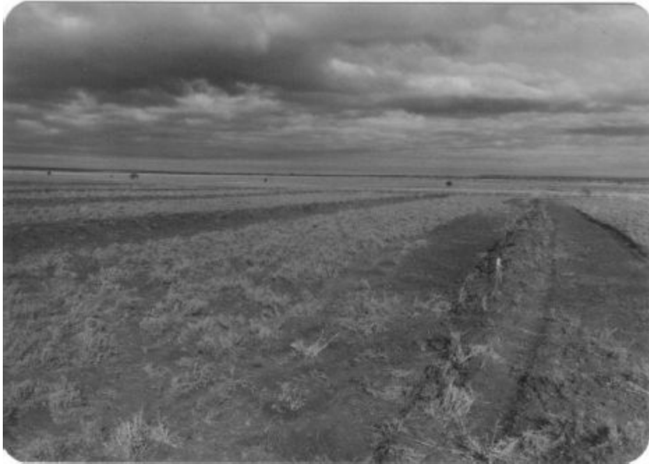
Plate 52 Finished steering banks. These two banks are close together as they channel water down the centre of a long ridge.
