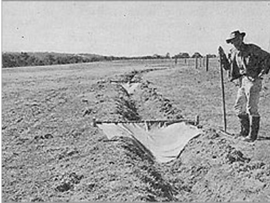
Plate 7 Early photo of irrigation flags in place awaiting the arrival of the water. 100mm (4") pipe us now used to span the channel.
