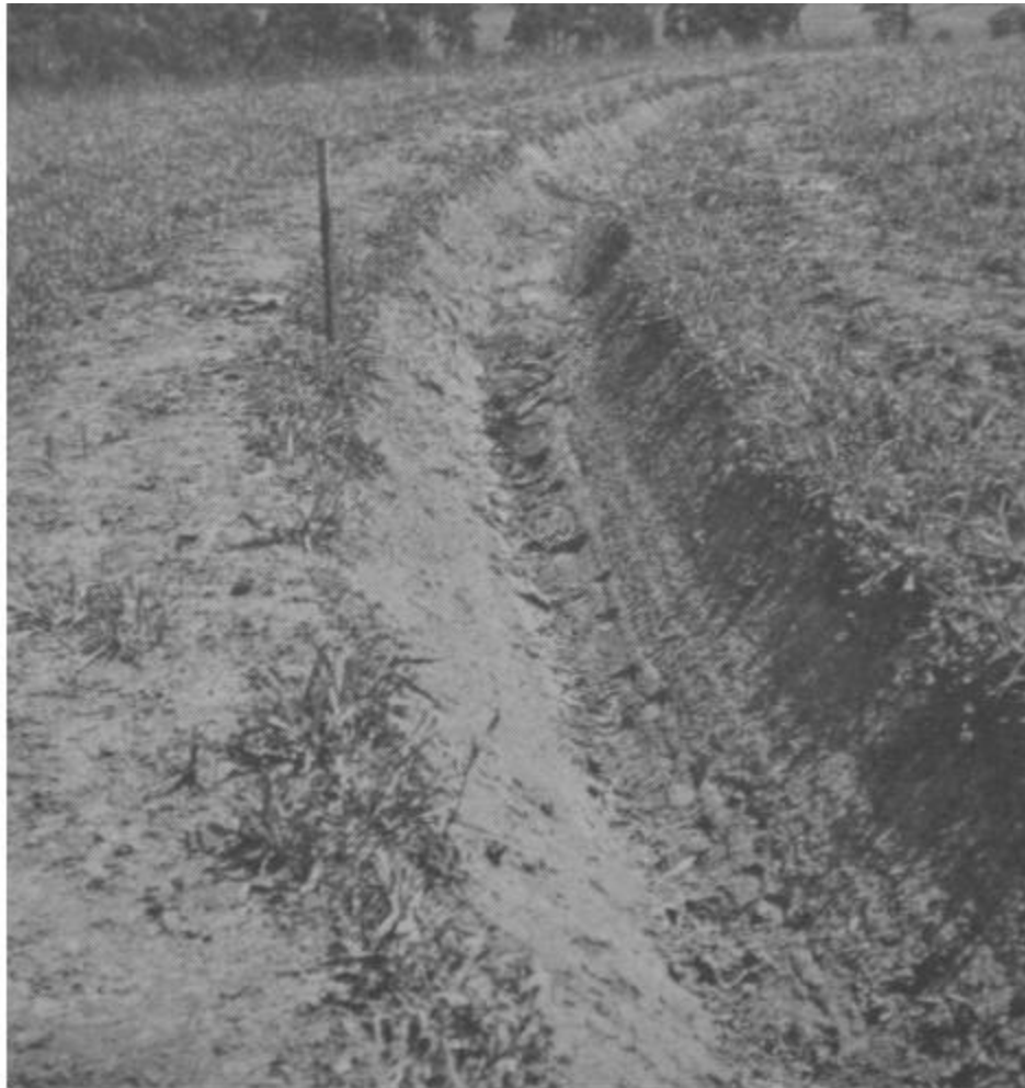
Plate 41 Close-up for an irrigation channel for Keyline Pattern (hillside) Irrigation. The channel is 1.2 m (48 inches) wide, and has a fall of 1 in 300. Note the relationship of the channel to the pegged line.
