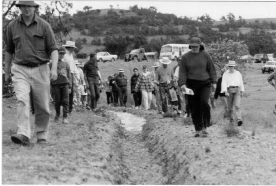
Plate 17 People follow the water as it appears to climbs out of the valley on its way to the irrigation area. Cars are along dam wall.
