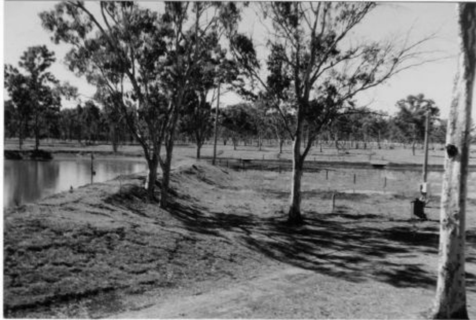
Plate 23 Panorama continuing from right side of plate 22. Flood-flow contour channel can be glimpsed wrapping around the dam in both photos. When full, the channel inundates back to the wall. Steering banks can be seen beyond the channel.
