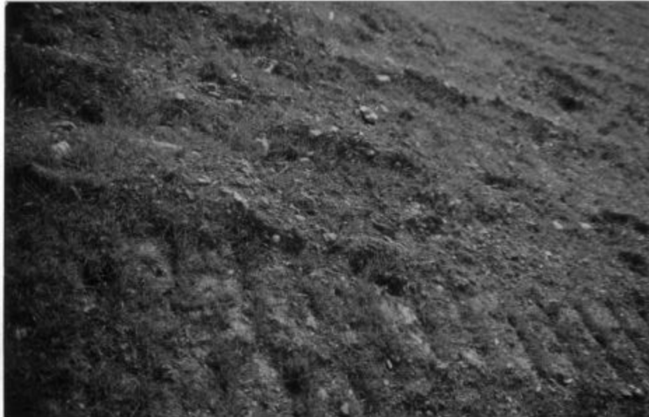
Plate 28 Grass is growing in the tack marks left by bulldozer in the topsoil on the batter slopes of the wall of a dam.
