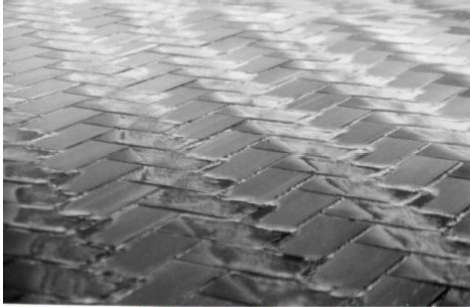
Plate 4 It doesn't take much to control shallow flowing water. This photo shows parallel streams of water flowing over a brick pathway. The water entered the area as a single stream but it was split up and controlled by the pattern in the brickwork. The flow is towards the camera.
