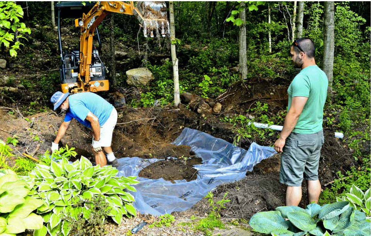
FIGURE 44 Building a bog. Hole is dug and lined with plastic, before being refilled with soil.
