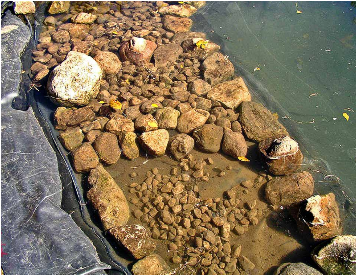
FIGURE 25 Partially completed planting shelves.
