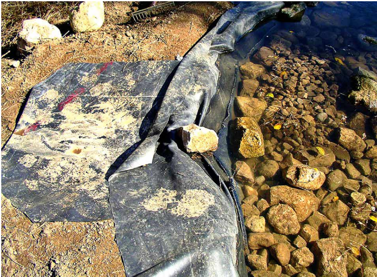
FIGURE 26 The spillway controls where overflow water will go.
