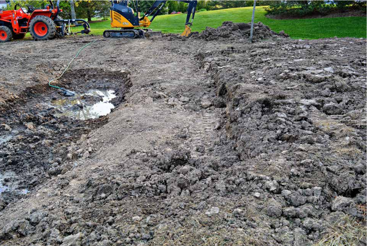
FIGURE 20 A pond that has been dug out. Notice the large planting shelf in the middle of the picture.
