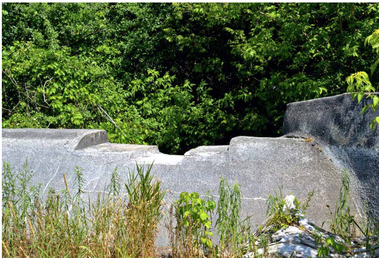
FIGURE 42 Concrete dam with outflow.
