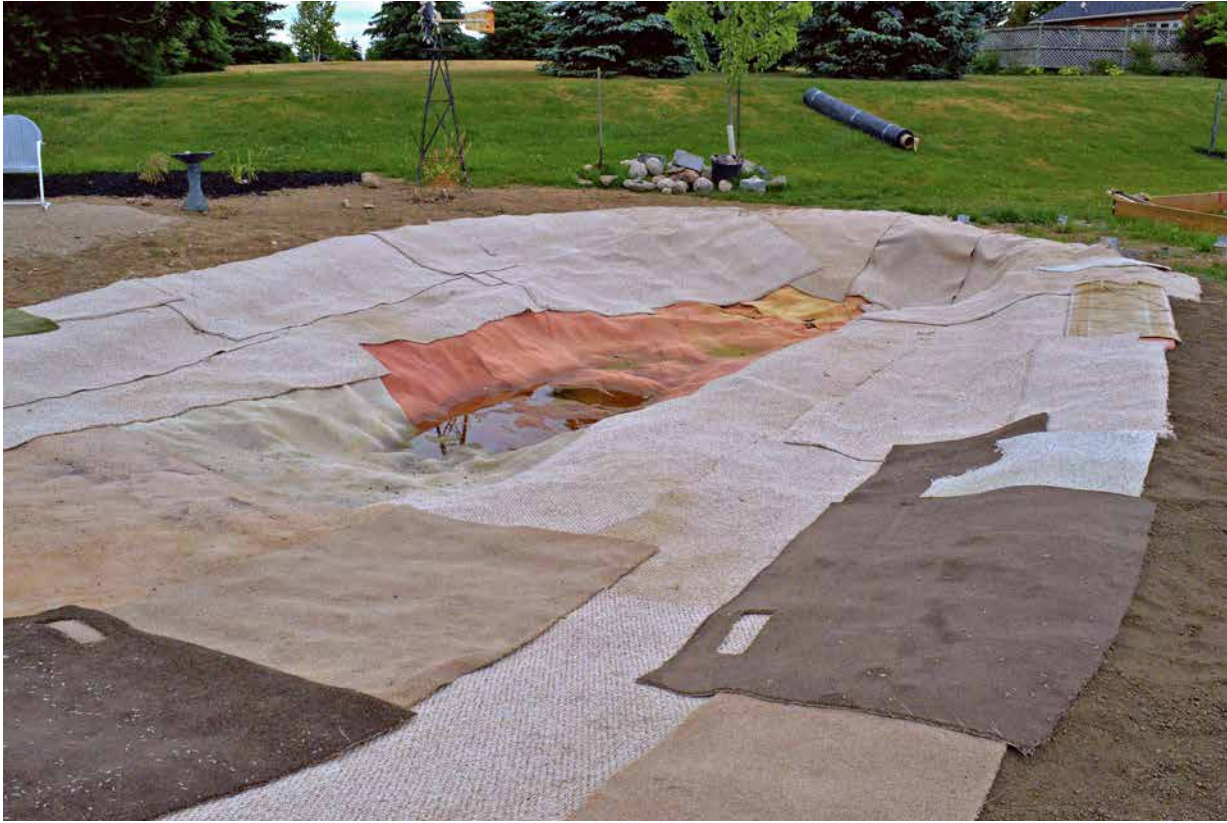
FIGURE 21 The carpet underlay will help protect the liner.
