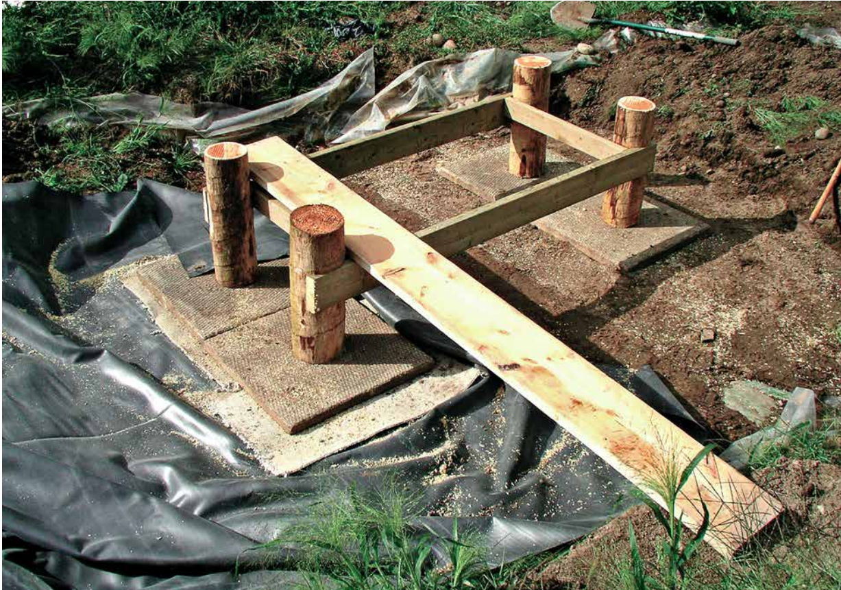
FIGURE 22 Footings for the bridge shown in figure 13.
