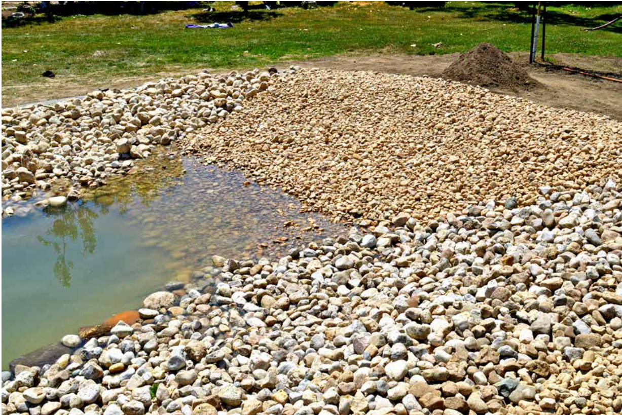
FIGURE 27 Beach area has been covered with smaller stones.
