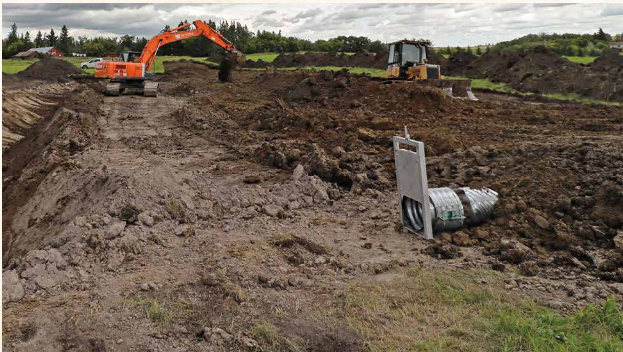
FIGURE 3.9. (top) The 150 mm (6 in.) swivel pipe going through the original dam wall. (bottom) The 400 mm (16 in.) flood pipe going through the newly constructed larger dam.
